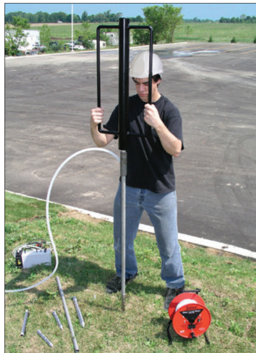
Installing Piezometers with a Manual Slide Hammer
